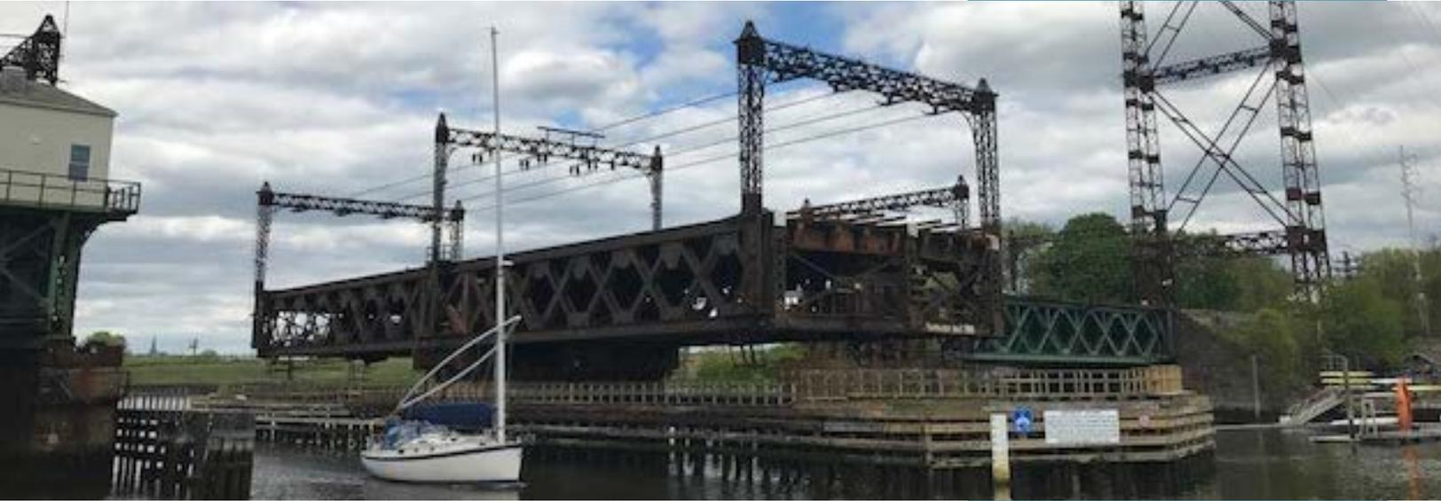
The existing Norwalk River Railroad Bridge (Walk Bridge), constructed in 1896, carries four railroad tracks and approximately 175 trains and 125,000 passengers daily. One of the oldest movable bridges on the Northeast Corridor, the 564-foot long, four span swing bridge has outlived its lifespan. The Walk Bridge has been subject to continued operational failures and vulnerable to damage from harsh weather conditions and requires replacement.
