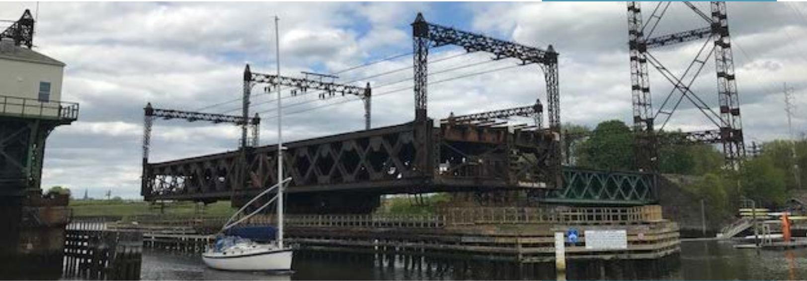
The existing Walk Bridge (Bridge No. 04288R, MP 41.5), constructed in 1896, carries four railroad tracks and approximately 200 trains and 125,000 passengers daily, with ridership that is projected to double by 2065. One of the oldest movable bridges on the Northeast Corridor, the 564-foot long, four span swing bridge has outlived its lifespan. The Walk Bridge has been subject to continued operational failures and vulnerable to damage from harsh weather conditions and requires replacement.
