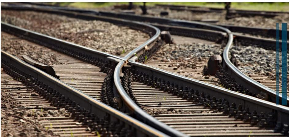
A **railroad switch** is a set of tracks that create a junction, that when moved allows for trains to change from one track to another.
