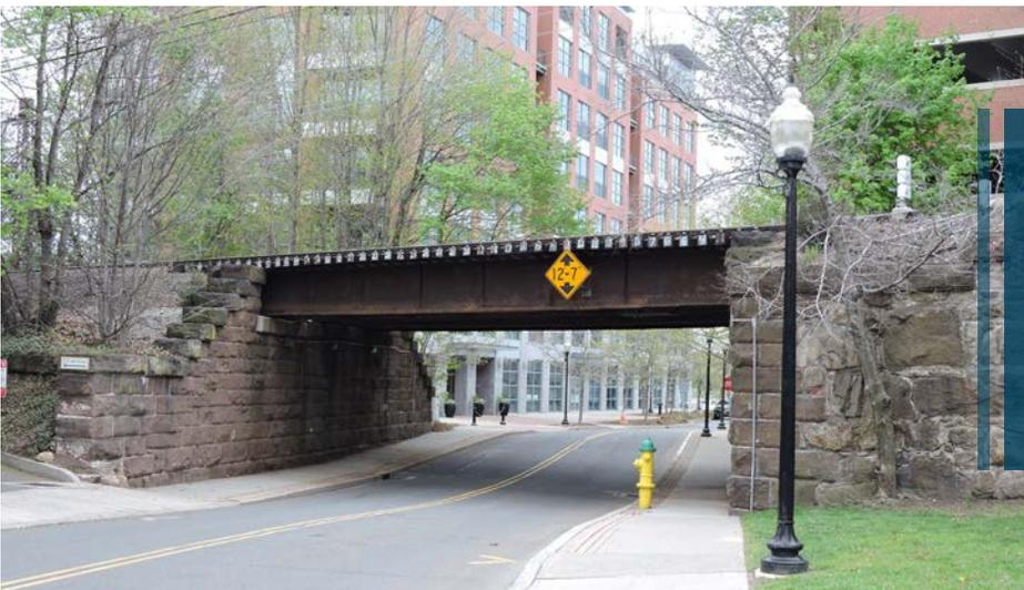
As part of the Danbury Branch Dockyard Project, the superstructure of the rail bridge over Ann Street will be replaced. This includes new weathering steel deck spans, new catenary systems and abutment wall improvements, which will maintain the 19th century character of the bridge.
