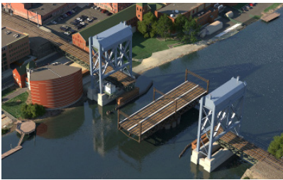
The existing swing span provides two navigation channels on either side of the center pivot pier.
