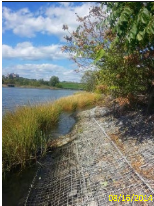
Photo 14 – Gabion slope along Norwalk River (looking north).
