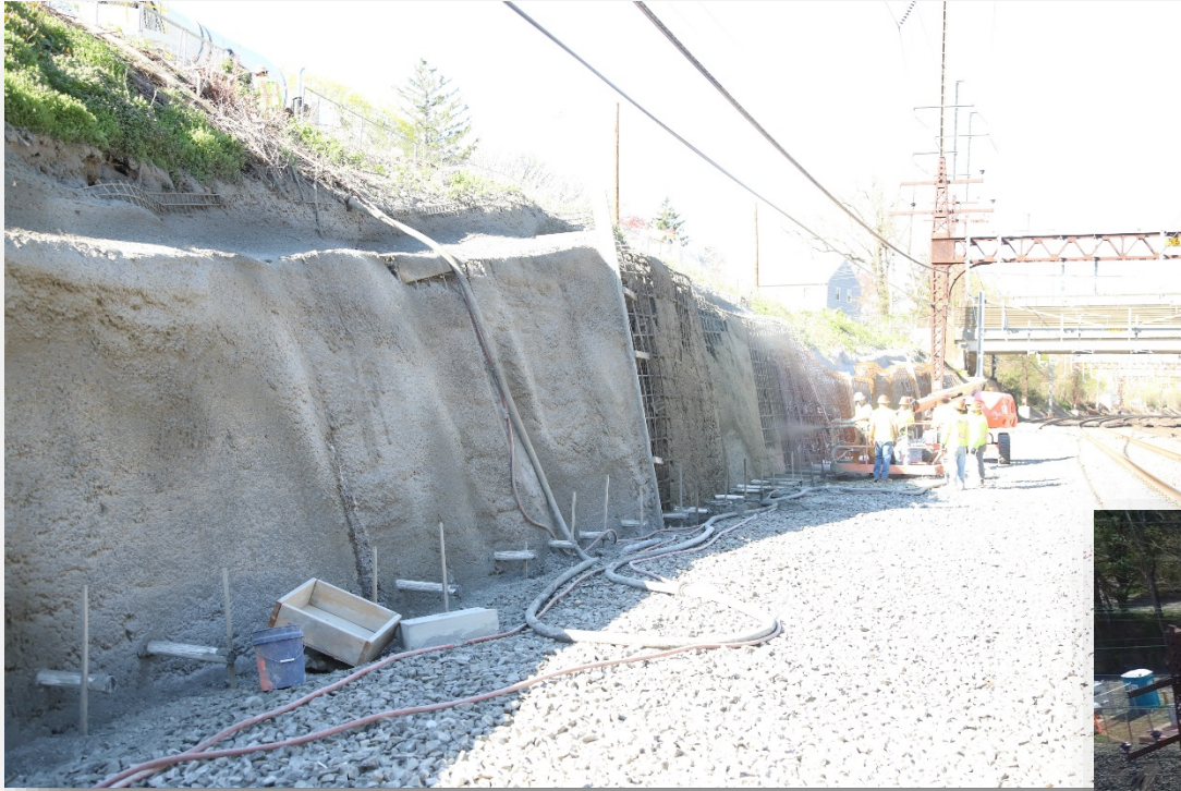
Shotcrete & Soil Nail Wall
