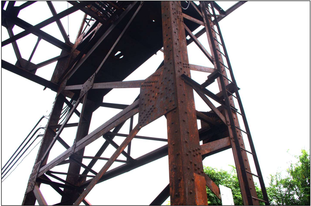
Photograph 10: East high tower (Bridge 530), detail of gusset plate and cross bracing, camera facing southwest.
