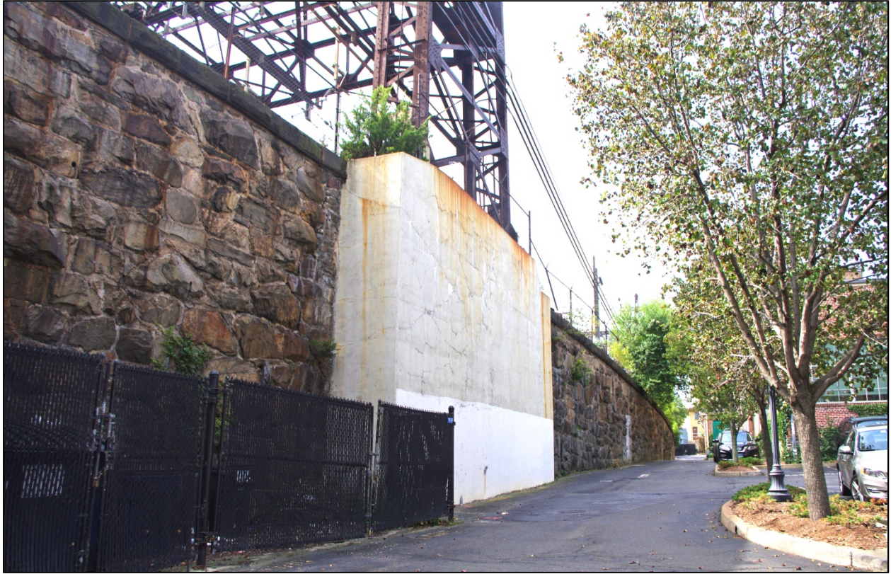
Photograph 19: North retaining wall and concrete base of west high tower (Bridge 529), camera facing southwest.
