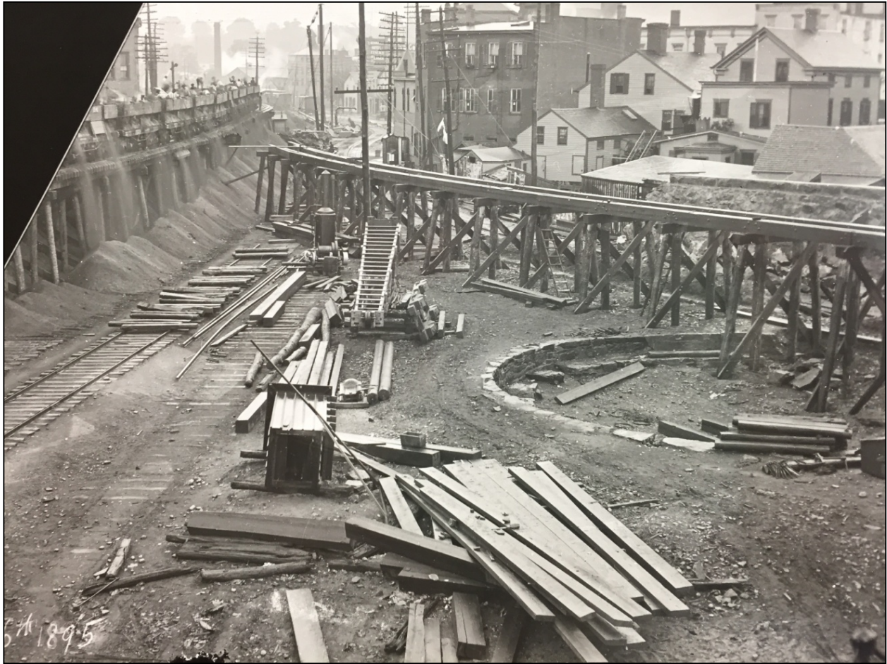
Figure 4: Dumping of fill for the embankment, South Norwalk, at the intersection of the main line (upper left), with trestle for creating the Danbury line embankment in the center, ca. 1895 (Norwalk History Room, Norwalk Public Library).
