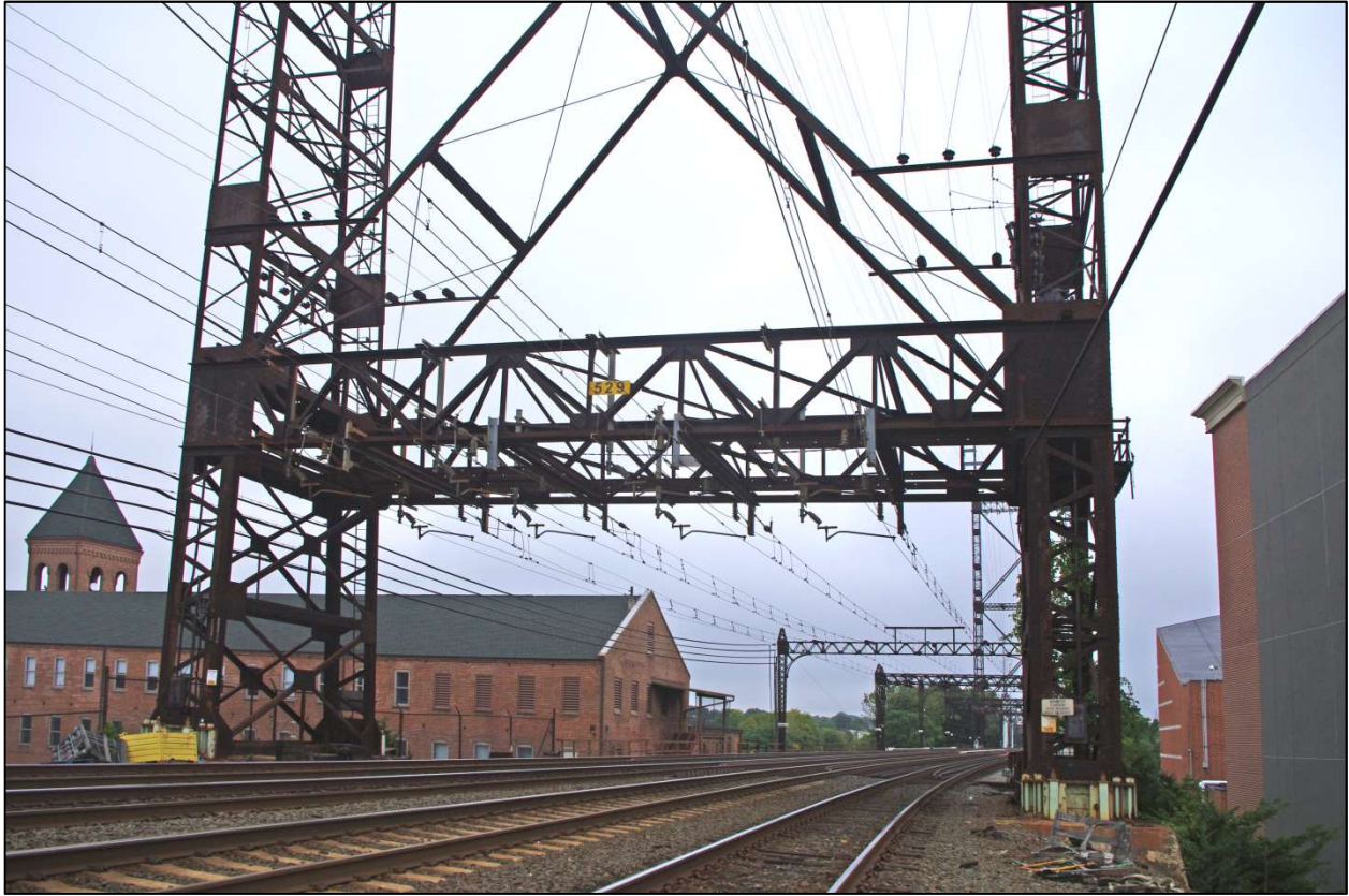
Photograph 7: West high tower (Bridge 529), detail of lowest cross-member, which also serves as a catenary support, camera facing northeast. Former Norwalk Iron Works, now the Maritime Aquarium, is visible in the background on the left.
