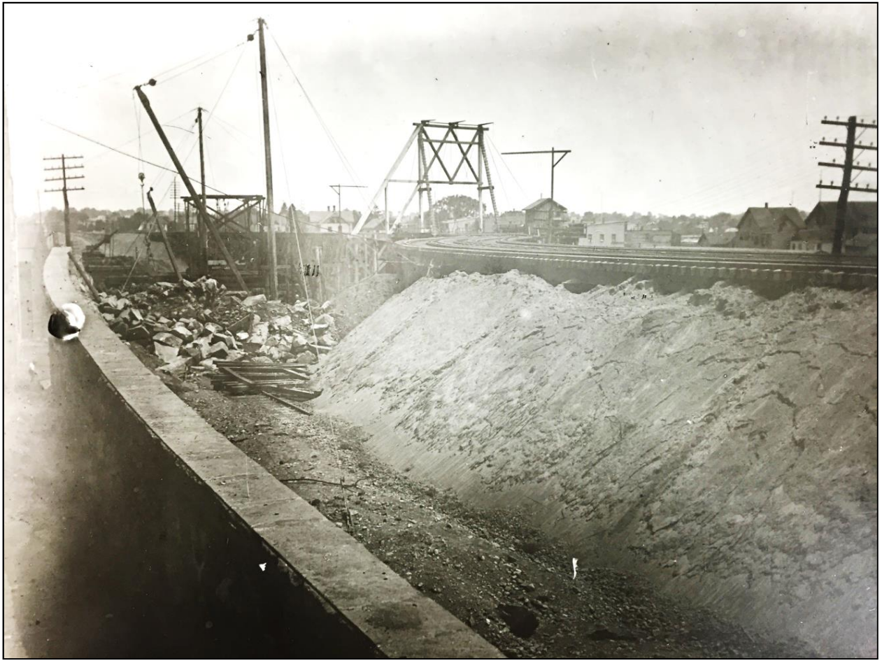
Figure 5: Completed retaining wall on the north side of the railroad right-of-way west of Water Street, ca. 1895 (Norwalk History Room, Norwalk Public Library). Fill for the embankment has been dumped from the trestle.
