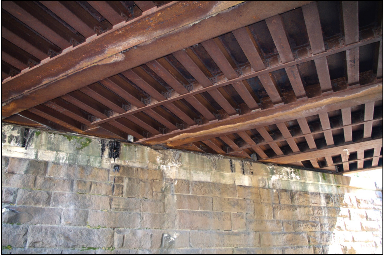
Photograph 29: Fort Point Street Railroad Bridge, detail of underside and east abutment, showing concrete bridge seat, camera facing southeast.
