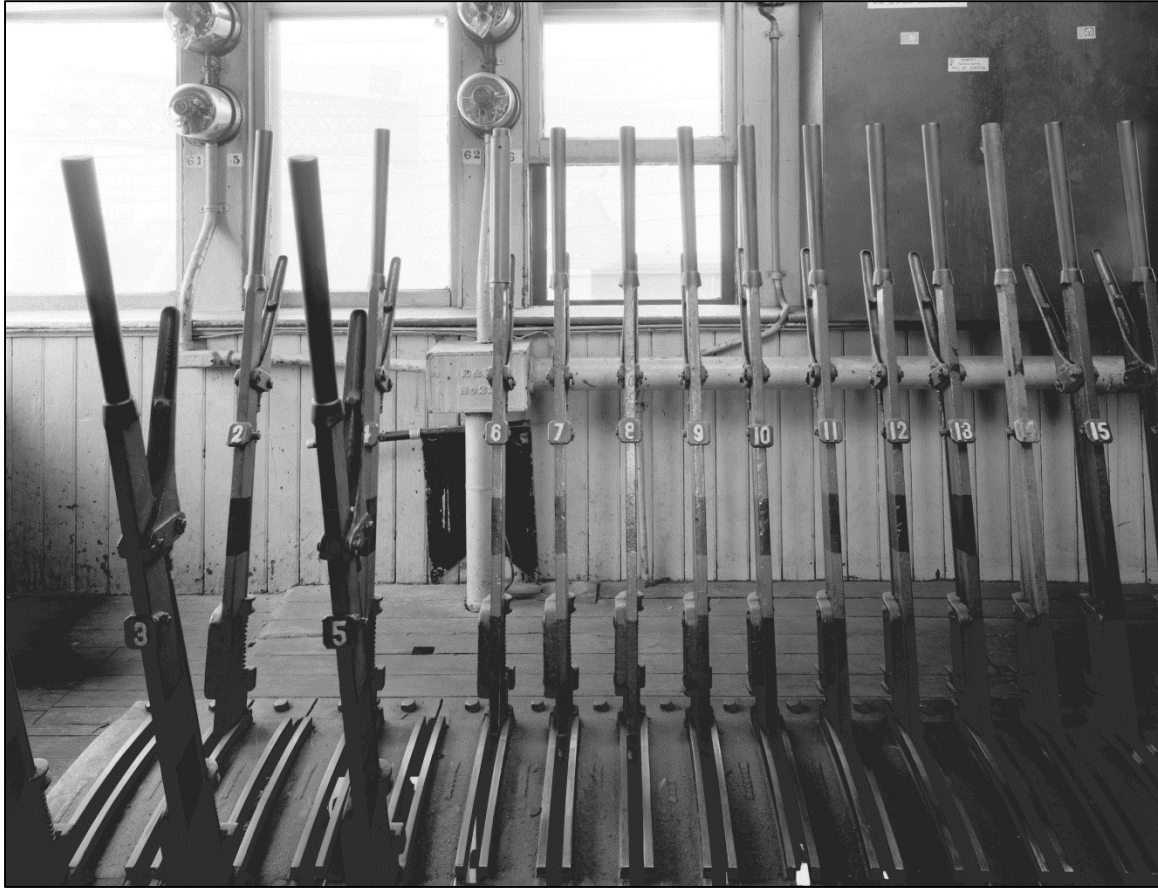
Figure 15: Interlocking tower (S.S. 44, South Norwalk Switch Tower Museum, 67 Washington Street), detail of switch levers, looking northwest, 1980 HAER photograph by Thomas Brown (CT-8-36).
