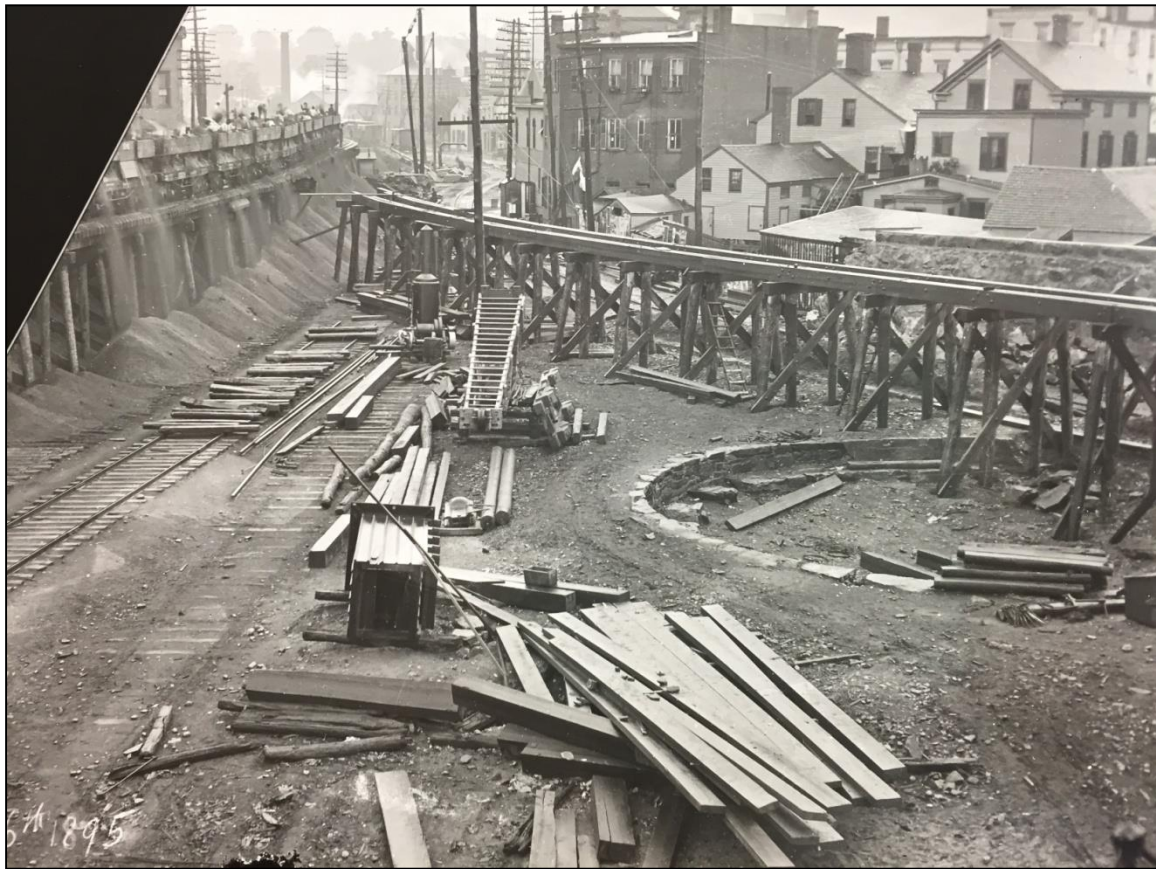
Image 1. View of four-tracking and elevation of the NY, NH & H line in 1895 (Norwalk History Room, Norwalk Public Library).
