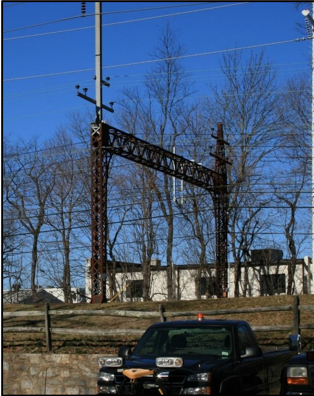
Photograph 1. Typical catenary bridge from the 1914 electrification.
