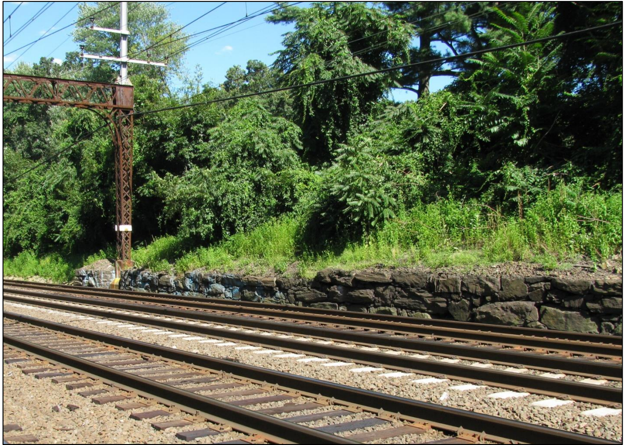
Photograph 19: Typical length of low stone retaining walls at the edge of the ROW.
